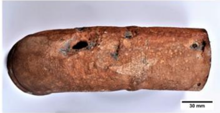
Figure 8: Large pits and perforations were seen on the surface of a steel pipe elbow. Credit: Kiani et al., 2019.
